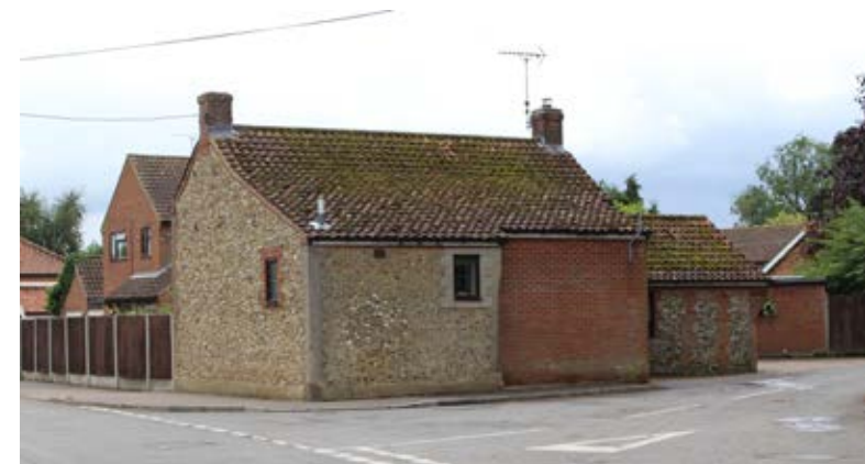
Cottage at Mill Street junction with Chantry Lane.
